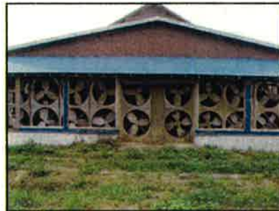
↑牛舎壁面の換気扇
